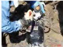
Corrosion protection (incl. Cathodic Protection) EPCC Basis
